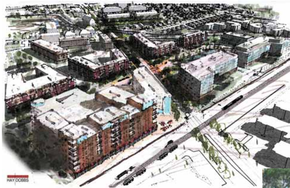
Blake Road Station looking Northeast at Blake Road and Excelsior Boulevard
