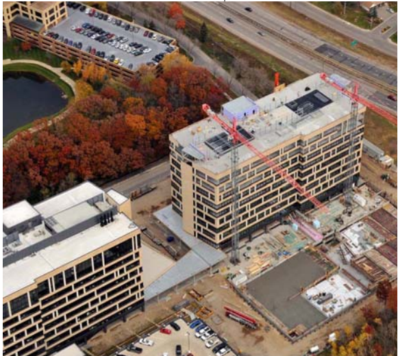
Opus Station Area: Phase 1 of the United Health Group office campus in Minnetonka is a 10-story, 350,000 square foot building completed in 2007. Phase 2 is currently under construction and will be another 10-story, 354,000 square foot building.
