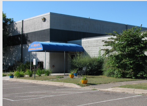
43 Hoops/County-owned development site
