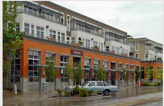
Mixed-use development with active street level uses
