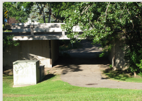
Existing trail underpass
